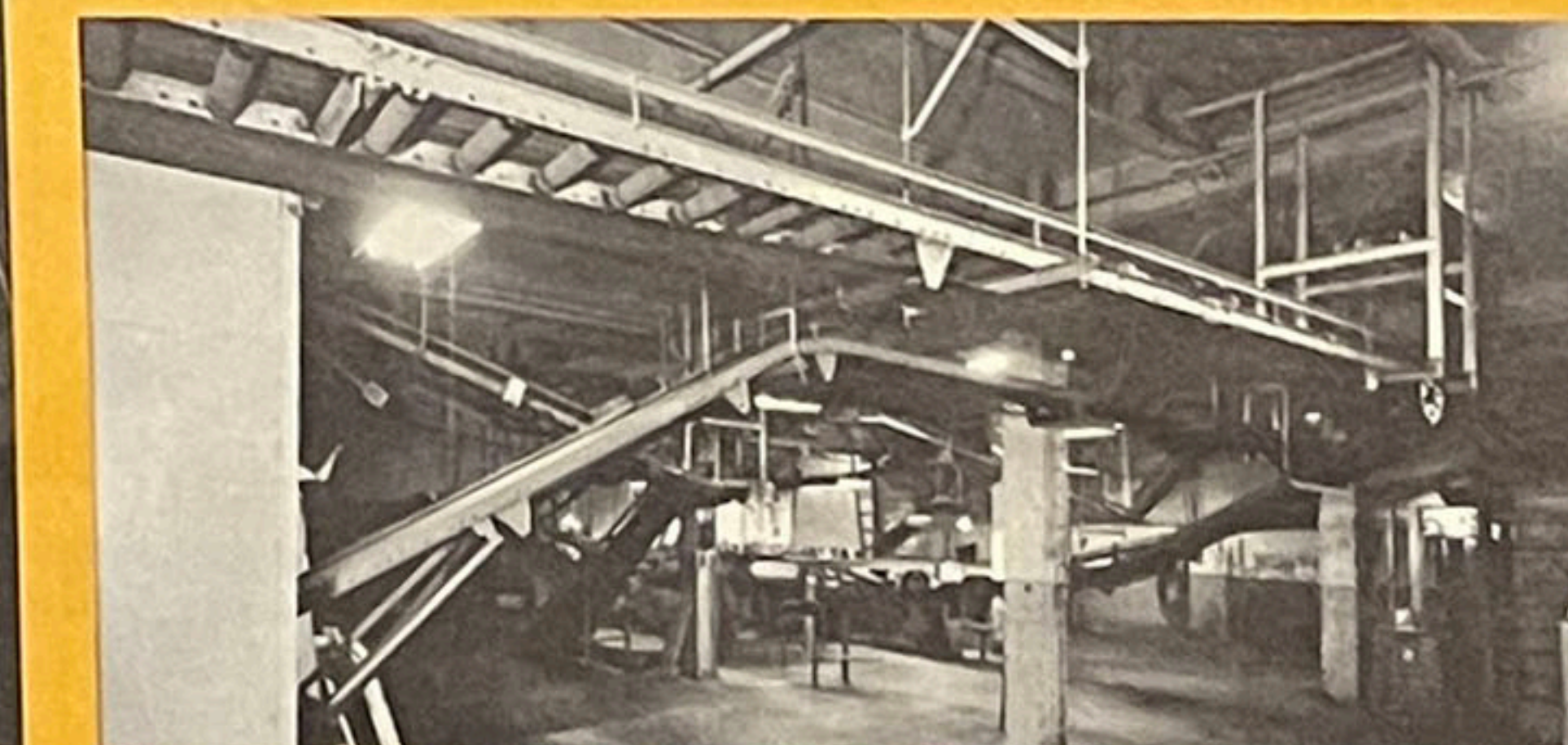
LINE 2—DECLINING BELT TO SOAKER, CASE UNLOADER TO CLEANER
